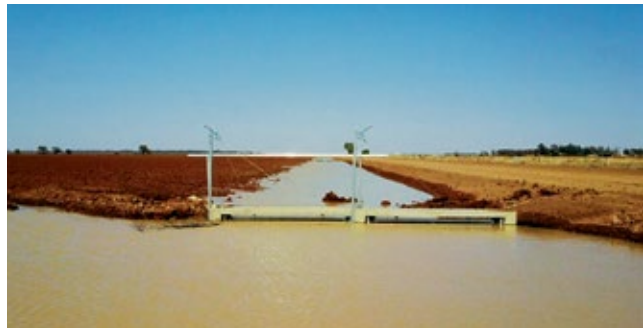
Figure 1: Head ditch structure – Padman Stops 2 x 1.5m.
