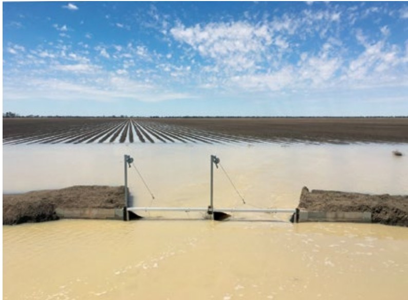
Water flowing from head ditch into distribution basin through twin outlets in Field 3.
