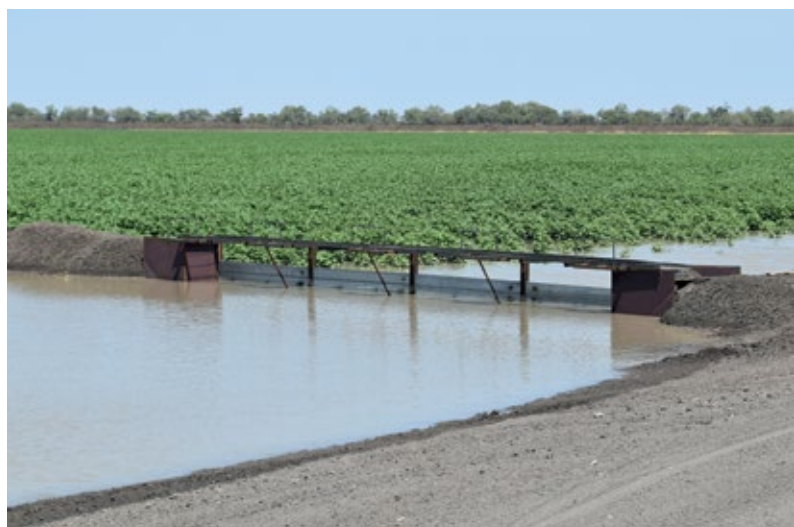
Figure 2: Head ditch weir.
