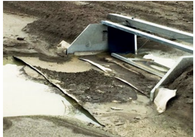
Tail drain structure of Field 3 with cement impregnated.
