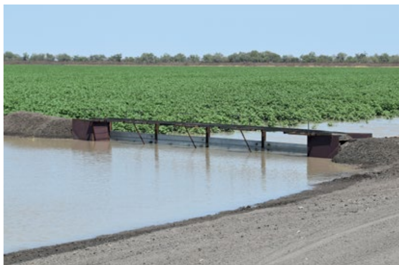
Figure 2: Head ditch weir.
